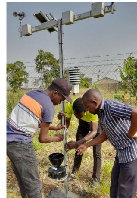
Putting finishes touches to an installed station in Palaro, northern Uganda
