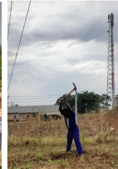
Clearing the ground for installation in Omoro district
