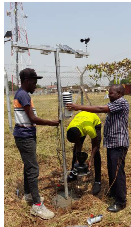
WIMEA-ICT team accompanied by Peter Natiko (right) from UNMA INSTALLING AN Automatic Weather station in Atiak
